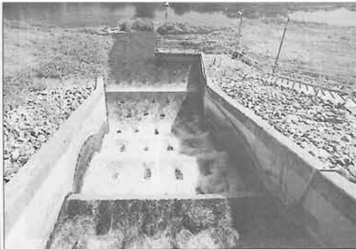
Treated water from the plant is emptied into the Codorus Creek in York, Pa. The plant's new limit is 0.8 parts per million of phosphorus. The water eventually reaches Chesapeake Bay.
