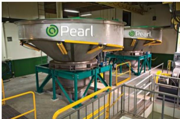
Ostara's Pearl system at Clean Water Services' Durham Advanced Wastewater Treatment Plant has been operating since June 2009 and is producing approximately one ton of slow release fertilizer per day.
